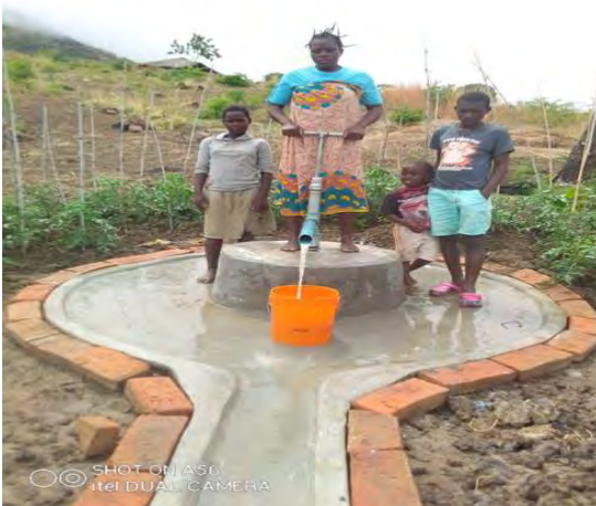
Left: A newly constructed well at Chakaka Village.
